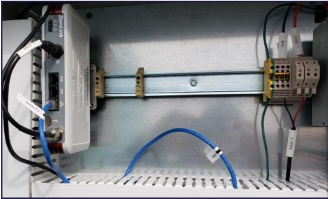
FreeWave's ZumLink IQ integrated with Inductive Automation's Ignition Edge MQTT installed at one of Sylvan Lake's field stations.
